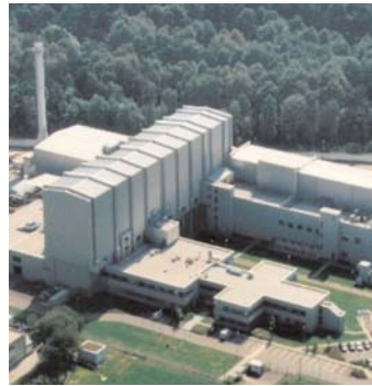
The ETW Plant in Cologne, Germany
