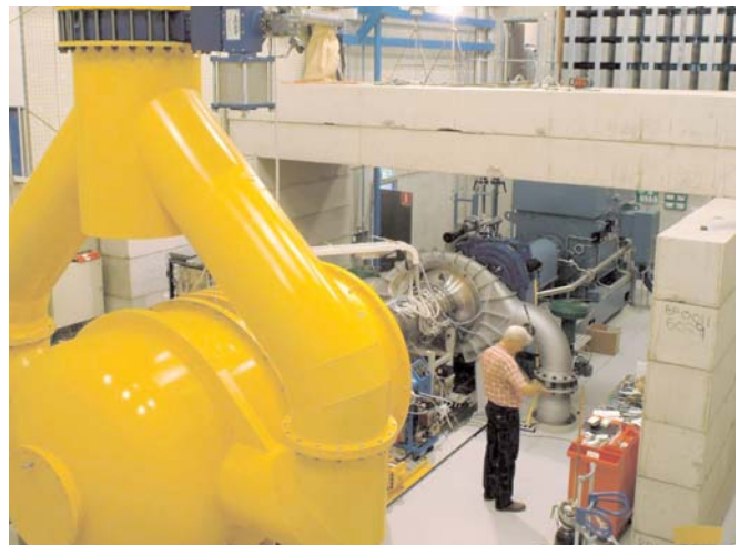
The New Turbomachinery Compressor Research Facility
